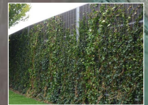
Ivy clad acoustic fencing - GREENSoundBlok Gramm Barriers Green Planting System or similar approved
